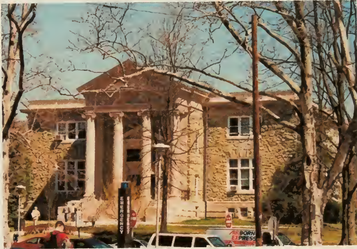
Photograph #41: The Library (1902-1904), now known as the Old Library, West Chester Normal School, now West Chester University, in West Chester Borough. The serpentine for this building came from Brinton's Quarry in Westtown Township.
